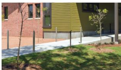
Permeable Paving Permeable paving is any system of pavers or porous material that allows for water to infiltrate into the ground. Pervious concrete allows water to pass through into the ground, reducing runoff.
