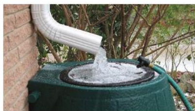
Rain Barrel and Cistern Rain barrels collect and store rainwater for non-potable usage, including landscape irrigation.
