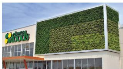
Green Walls A green wall is a vegetated wall, which can provide shade and lower cooling costs.
