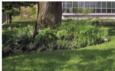
Bioswale Around Existing Tree A bioswale is a landscaped feature with sloped sides that conveys water and allows it to infiltrate into the ground.
