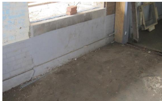
Application of Impermeable Coating
